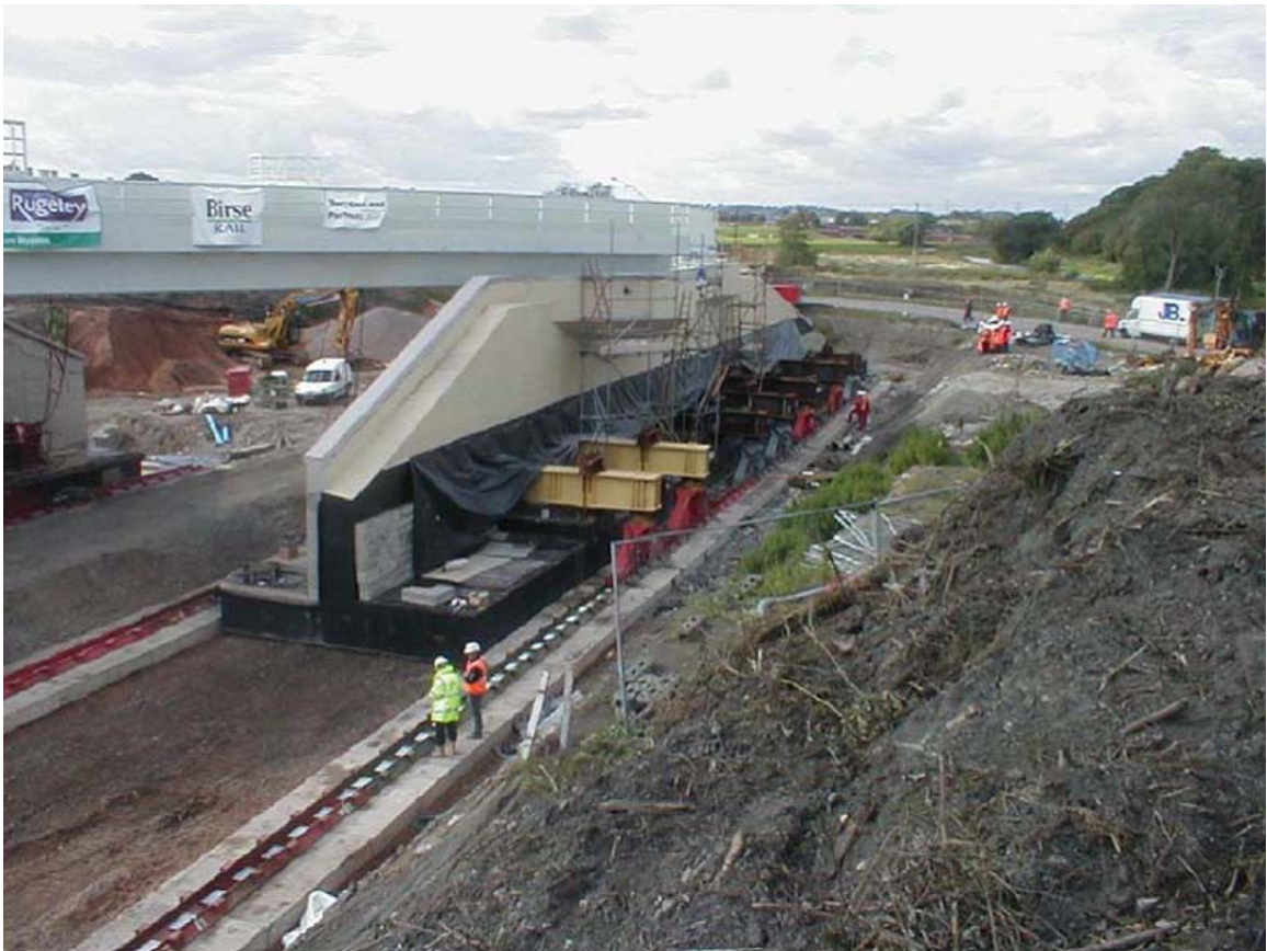
Rugeley Bridge Slide
